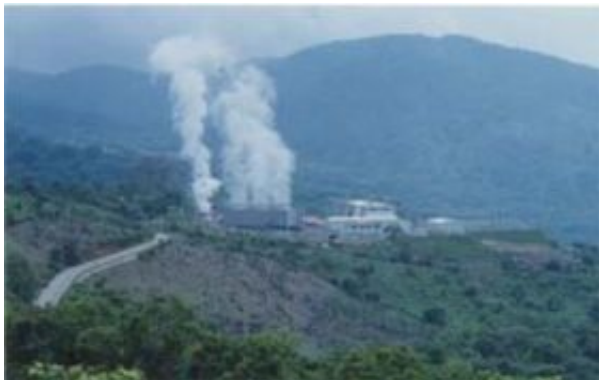
Geothermal power plants harness energy created by heat at the Earth's core. Credit: Dina Lopez/Ohio University
