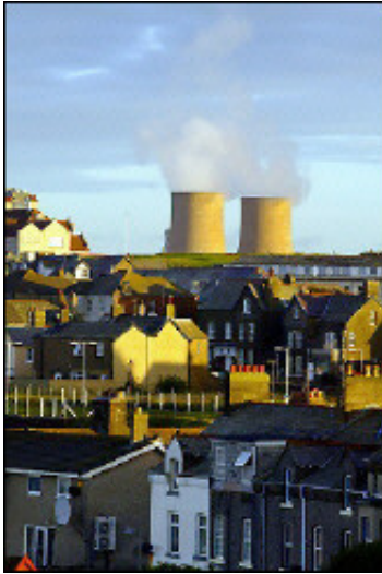
Steam rises from cooling towers at the Sellafield nuclear plant in northern England
