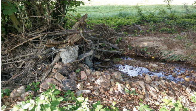
Woody debris clogging a small creek of the Ahr river, leading to temporal ponding, massive sediment deposition and overbank spillways of the flood water. Credit: M. Dietze, GFZ
