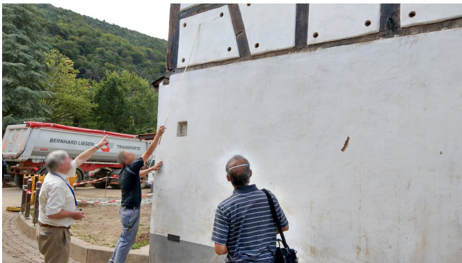
Owner showing the water level of the 14 July flood on his house in Walporzheim. Note the 2.2 m water mark of the 1804 flood and the 0.6 m mark from 2016 for comparison. Credit: Michael Dietze, GFZ
