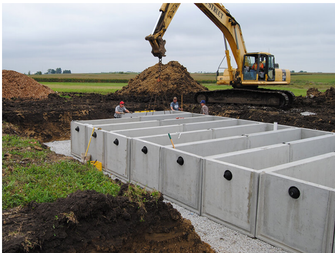
Contractors place concrete bioreactor liners into the trench. Credit: Michelle Soupir
