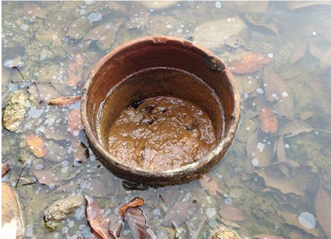
Bubbles of methane gas in water around an unplugged oil/gas well in Pennsylvania. Credit: Mary Kang
