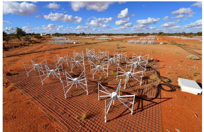
Antennas of the Murchison Widefield Array (MWA) low-frequency radio telescope. Credit: Dragonfly Media, Author provided
