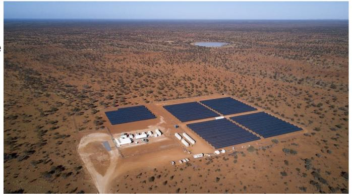
Aerial view of the MRO power station, which has an array of 5,280 solar panels and battery with RFI shielding.
