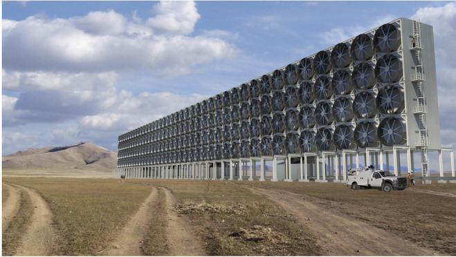
This illustration provided by Carbon Engineering in October 2018 shows one of the designs of the company's air contactor assemblies to remove carbon dioxide from the atmosphere. More than a 100 countries—responsible for about two-thirds of the world's heat-trapping gases—have announced plans to cut their greenhouse gas emissions to "net zero" in coming decades to help curb man-made climate change. (Carbon Engineering via AP)
