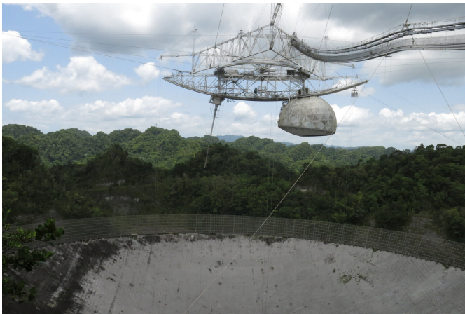
This July 13, 2016 file photo shows one of the largest single-dish radio telescopes at the Arecibo Observatory in Arecibo, Puerto Rico. Giant, aging cables that support the radio telescopes are slowly unraveling in this U.S. territory, threatening scientific projects that researchers say can't be done elsewhere on the planet. (AP Photo/Danica Coto, File)
