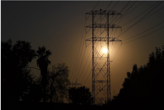
Electrical power lines are seen in Los Angeles on August 19, 2020 during a triple-digit heatwave
