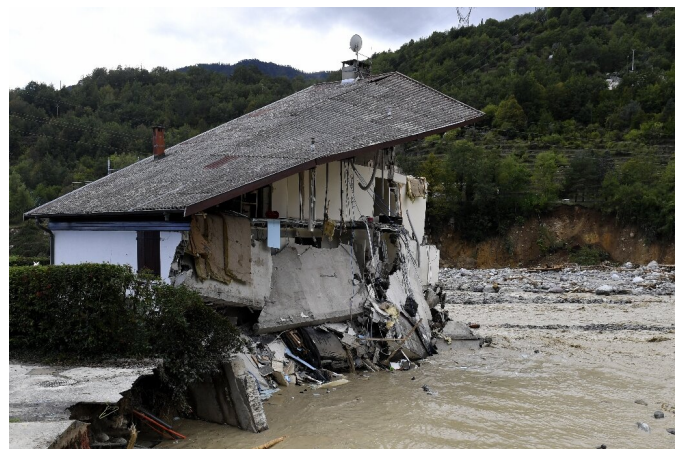
A house destroyed by floodwaters in Roquebilliere, southeastern France
