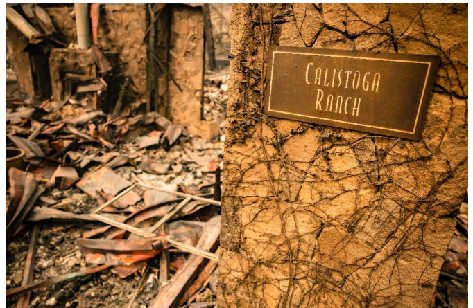
The rubble that was once the main building at Calistoga Ranch is pictured following damage by the Glass Fire
