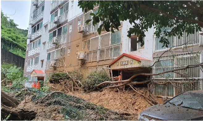
A landslide hit this apartment building in Geoje, South Korea after slamming southern Japan with record winds and heavy rains
