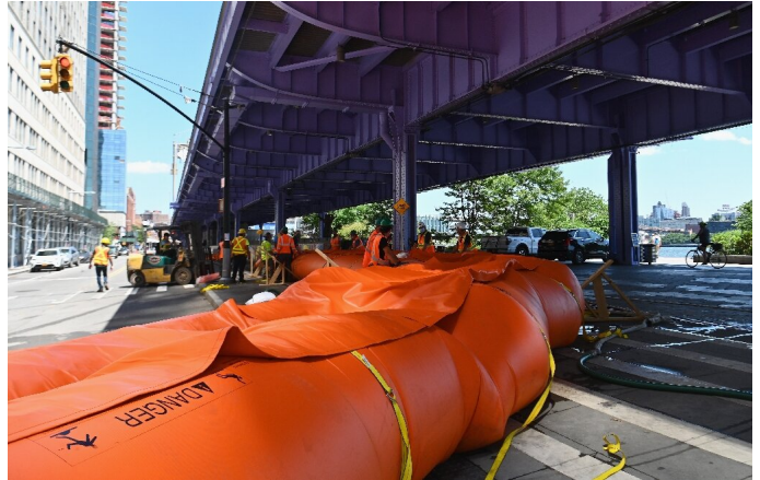
Workers set up temporary plastic flood barriers and sandbags known as 'Tiger Dams' in lower Manhattan to protect the area from flooding as tropical storm Isaias approaches New York City on August 3, 2020
