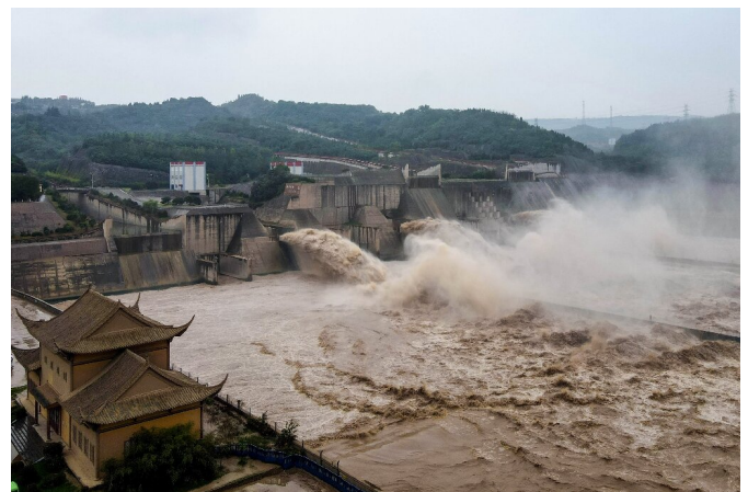
Dams such as the Xiaolangdi Reservoir in Luoyang, central Henan province, have opened sluice gates to release upstream water pressure
