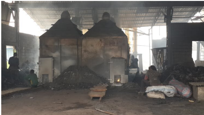
A typical lead battery recycling plant without adequate pollution controls. Credit: Occupational Knowledge International
