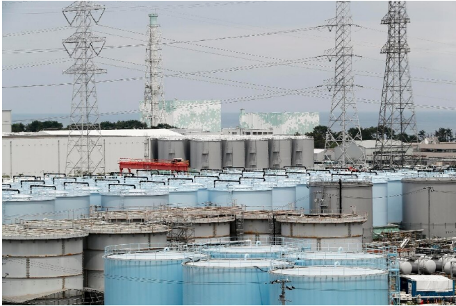
Storage tanks holding radioactive water at Japan's crippled Fukushima power plant
