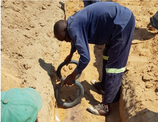
Farmers install SWRT membranes in Marange area of Zimbabwe as part of the technology's first trial in Africa in September 2019. Credit: N. Chirinda / CIAT
