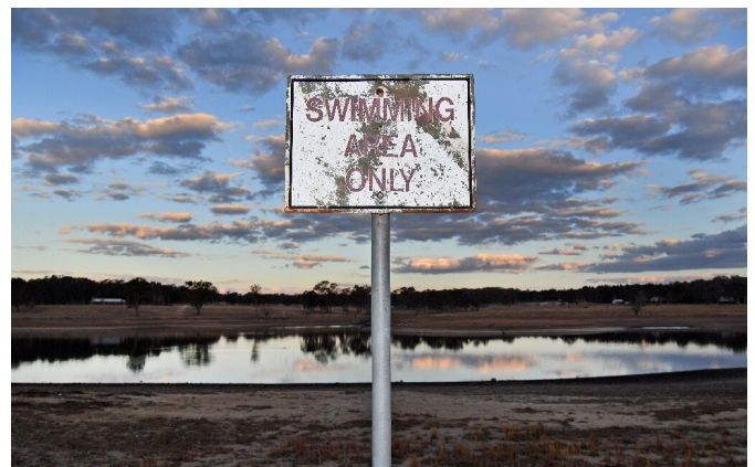
Storm King dam near Stanthorpe in regional Queensland used to be a popular swimming spot, but there is hardly any water left now
