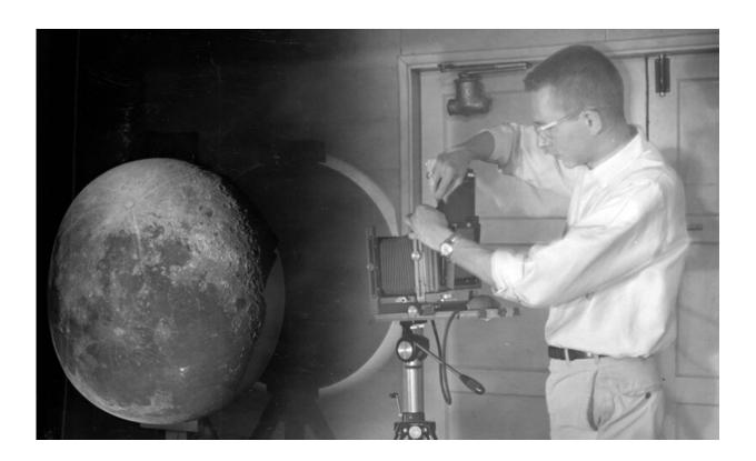
William Hartmann projected photographic plates of the moon onto a white hemisphere to create the Rectified Lunar Atlas. Credit: UA Lunar and Planetary Laboratory
