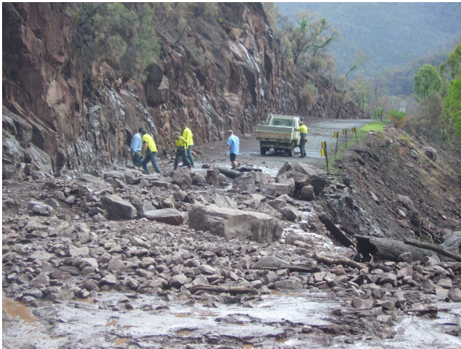
Debris flow can damage roads and infrastructure. Credit: Adrian Murphy (Melbourne Water)
