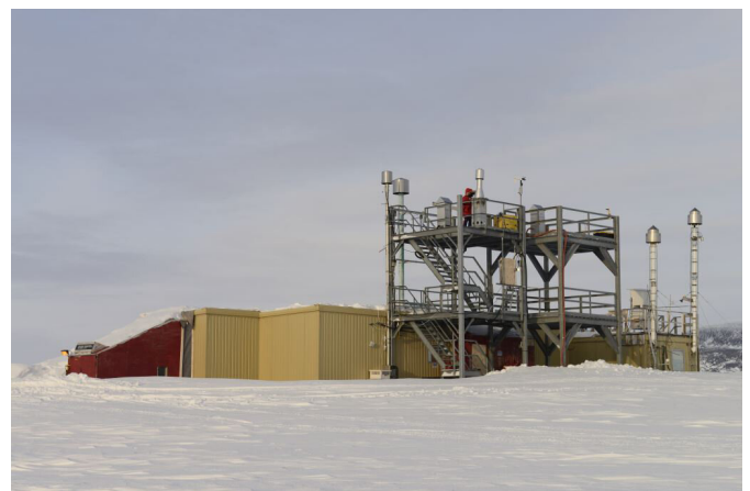
The Dr. Neil Trivett Global Atmosphere Watch (GAW) Observatory is the most northerly site in the global network, located at Alert, Nunavut, Canada (approximately 800km south of the geographic North Pole). Environment and Climate Change Canada operates the observatory, which hosts research campaigns and facilitates long-term measurements of a
