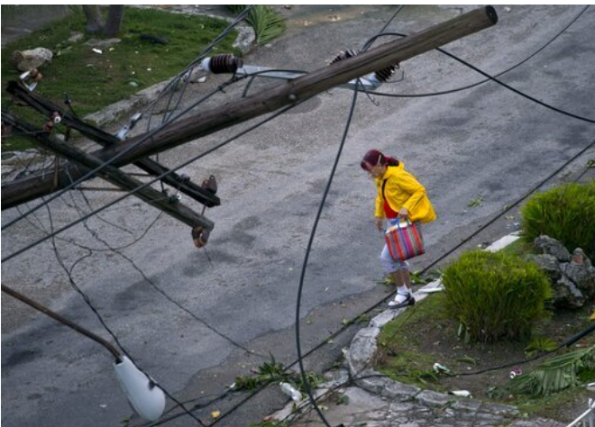
A woman walks under a lamp post toppled by a tornado in Havana, Cuba, Monday, Jan. 28, 2019. A tornado and pounding rains smashed into the eastern part of Cuba's capital overnight, toppling trees, bending power poles and flinging shards of metal roofing through the air as the storm cut a path of destruction across eastern Havana. (AP Photo/Ramon Espinosa)
