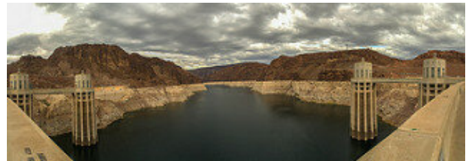
The water surface elevation of Lake Mead has dropped about 15 metres from its highest level, revealing a white ring of mineral deposits on its walls. Credit: Wayne Hsieh/flickr , CC BY-NC
