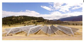
The CHIME telescope incorporates four 100-metre long U-shaped cylinders of metal mesh that resemble snowboard half-pipes, with total area equivalent to five hockey rinks. CHIME reconstructs the image of the overhead sky by processing the radio signals recorded by thousands of antennas. Its signal processing system is the largest of any telescope on Earth, allowing it to search huge regions of the sky simultaneously. Credit: CHIME
