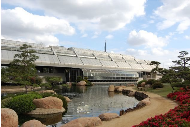
The Tillman Water Reclamation Plant in Van Nuys treats 80 million gallons of wastewater per day. Credit: Wikimedia Commons
