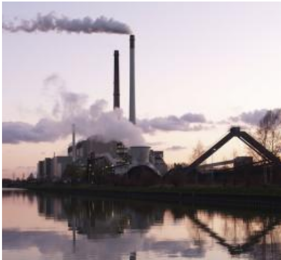
A coal power plant in Datteln, Germany, that transforms chemical energy into 36%-48% electricity and the remaining 52%-64% into waste heat. Image credit: Arnold Paul. Wikimedia Commons.
