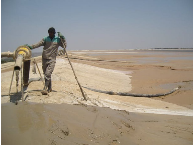
A gold tailings dam under construction in South Africa. Author supplied
