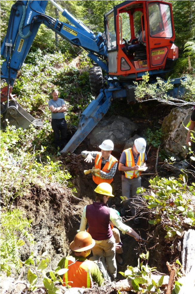
The team inspecting the trench during initial opening. Credit: Kristin Morell
