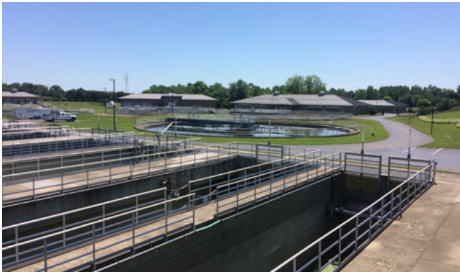
Alum Creek Waste Water Reclamation Facility. Credit: Ohio University
