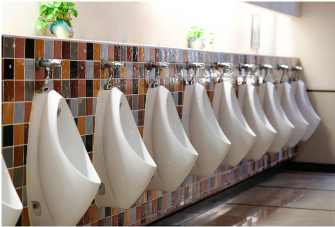
Urinals need less space than cubicles, so more men can use the toilet at the same time. Credit: shutterstock.com
