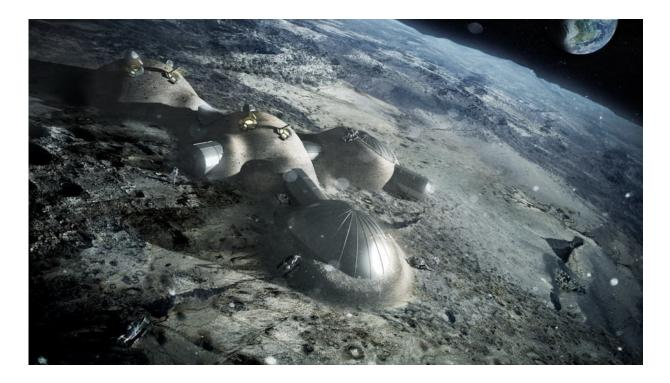
Artist's concept for a multi-dome lunar base, which would be constructed by 3Dprinting robots using lunar dust (regolith). Credit: ESA/Foster + Partners
