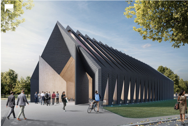
The Longhouse, a prototype 'mass timber' building designed by an MIT class, demonstrates that even huge buildings can be built primarily with wood. Credit: MIT Mass Timber Design
