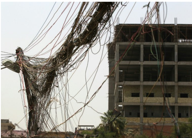
A picture taken on July 26, 2018, shows loose wires coming from a generator in Baghdad installed to supplement the poor public power grid
