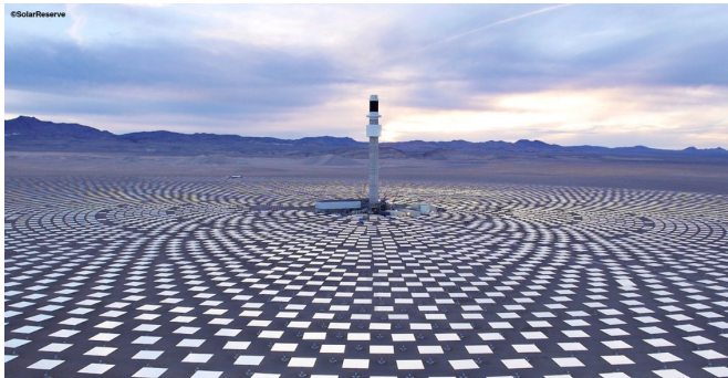
Crescent Dunes CSP project with 10 hours of storage. Credit: SolarPACES
