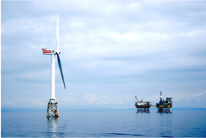
Offshore wind turbine near Scotland. Credit: U.S. Department of the Interior
