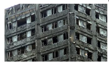
The flammable cladding was instrumental in the fire spreading so quickly. Credit: Flickr/ChiralJohn, CC BY
