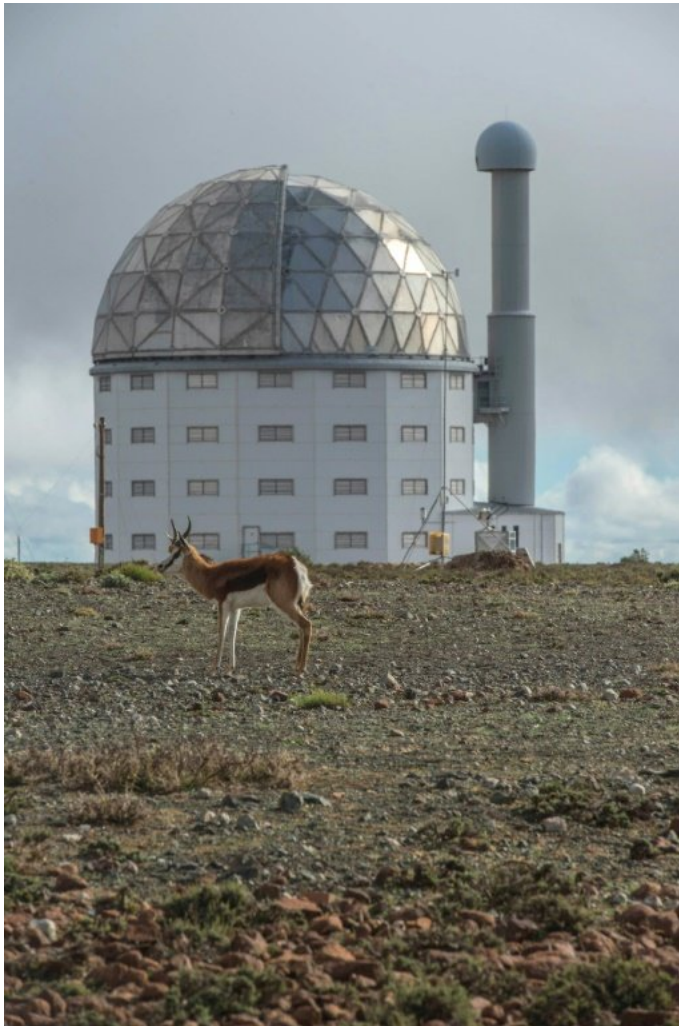
The optical telescope is housed in a white dome-shaped building made of carbon fibre to protect it against temperature fluctuations in the Karoo desert
