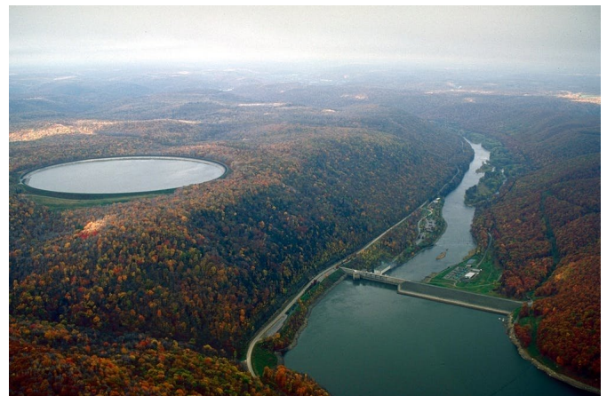
The Seneca pumped storage reservoir, on the left, and the Kinzua Dam on the Allegheny River in Warren County near Warren, Pa. Credit: U.S. Army Corps of Engineers Digital Visual Library
