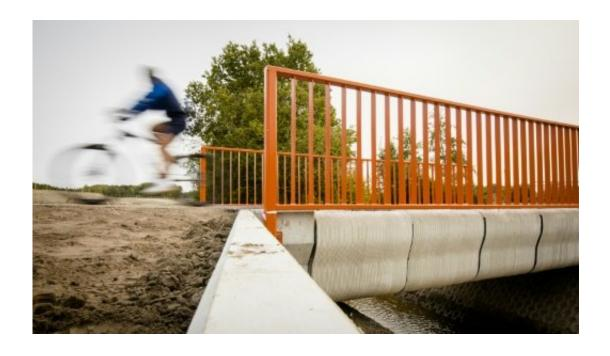
A 3D printer laid some 800 layers of concrete to create the eight-metre bicycle bridge in the Dutch town of Gemert
