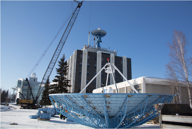
The new AS-2 antenna stands atop the Elvey building at the University of Alaska Fairbanks. In the foreground rests the old AS-2 antenna it replaced. Credit: Jeff Beiderbeck/PWP Photography
