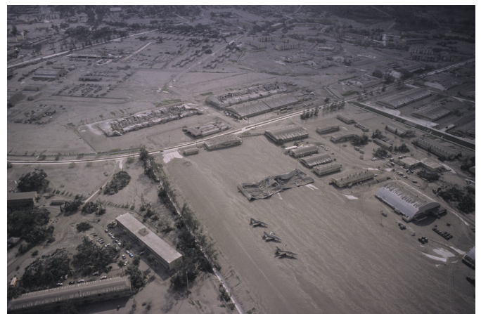
Damage from volcanic ash at Clark Air Force Base in the Philippines after the June 15, 1991, eruption of Mount Pinatubo. Credit: Richard Hoblitt/U.S. Geological Survey
