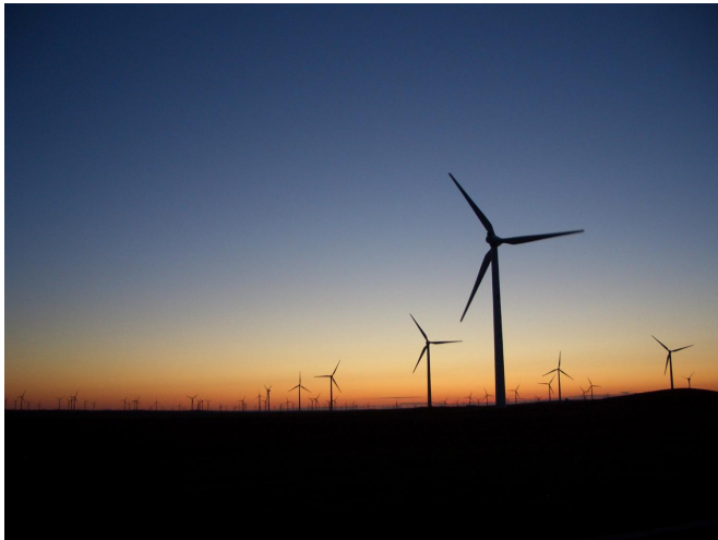
Large-scale wind power plant in China. Credit: Wenzhu Hou, distributed via imaggeo.egu.eu. This image is distributed under a Creative Commons Attribution licence.
