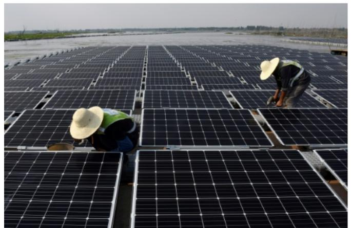
The 40-megawatt power plant has 160,000 panels resting on a lake that emerged after the collapse of a coal mine in central Anhui province
