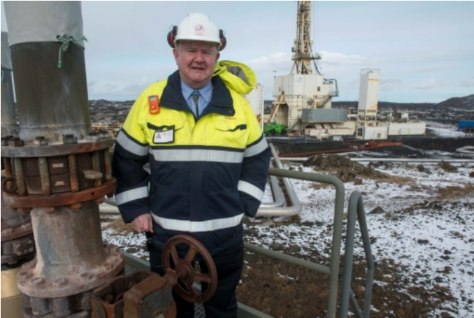
Engineer Albert Albertsson says Iceland's geothermal well could generate five to 10 times more power than a conventional well
