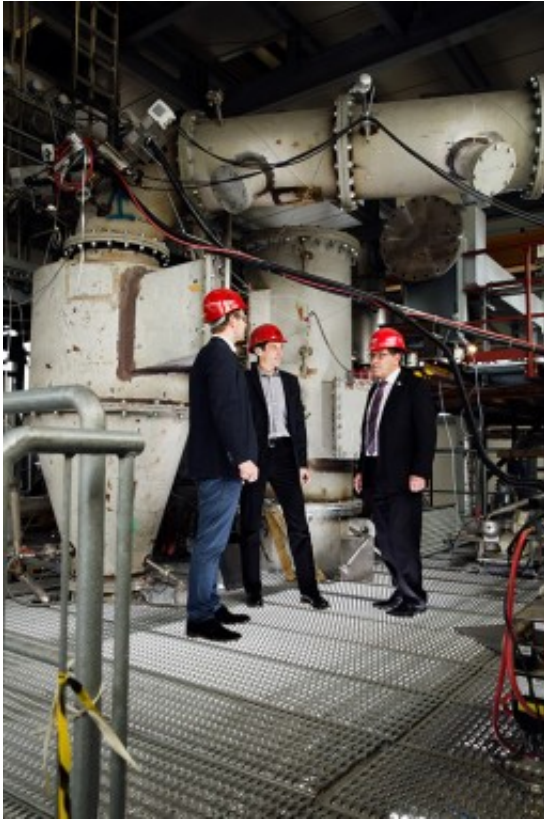
Jochen Hiltz, Dr.-Ing. Jochen Ströhle, Prof. Dr.-Ing. Bernd Epple (from left to right) in the CO 2 testing facility, which houses the 1 MW experimental pilot plant. Credit: Katrin Binner
