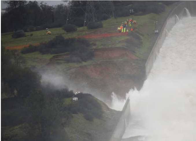
Water flows through break in the wall of the Oroville Dam spillway, Thursday, Feb. 9, 2017, in Oroville, Calif. Engineers don't know what caused what state Department of Water Resources spokesman Eric See called a "massive" cave-in that is expected to keep growing until it reaches bedrock. (AP Photo/Rich Pedroncelli)
