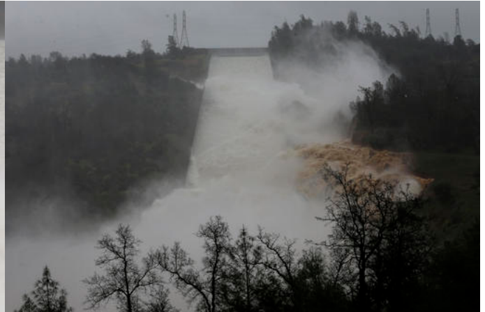
Water rushes down the Oroville Dam spillway, Thursday, Feb. 9, 2017, in Oroville, Calif. State engineers on Thursday discovered new damage to the Oroville Dam spillway, the tallest in the United States, though they said there is no harm to the nearby dam and no danger to the public. Earlier this week, chunks of concrete went flying off the spillway, creating a 200-foot-long, 30-foot deep hole. (AP Photo/Rich Pedroncelli)
