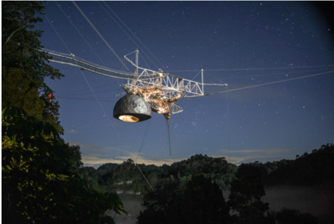
The suspended support platform of radio receivers at Arecibo Observatory in Puerto Rico. Credit: USRA
