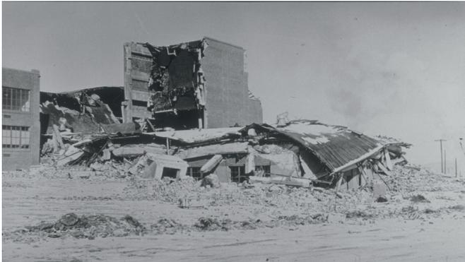
A photograph of damage to Helena High School, which collapsed following a major aftershock of the 1935 Helena magnitude 6.2 earthquake in Montana. Credit: NOAA National Geophysical Data Center
