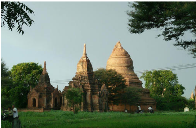
This photo provided by David Greco/@daveinosaka shows a temple in Bagan, Myanmar, shortly after it was damaged by a powerful earthquake that shook central Myanmar on Wednesday, Aug. 24, 2016. The earthquake, measuring a magnitude 6.8, damaged scores of ancient Buddhist pagodas in Bagan, a major tourist attraction, officials said. (David Greco/@daveinosaka via AP)
