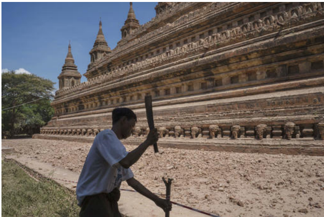
A man nails a stake to set up a security perimeter around earthquake effected Sitanagyi Pagoda in Bagan, Myanmar, Thursday, August 25, 2016. Workers surveyed the damage Thursday after a powerful earthquake shook Myanmar Wednesday, damaging a number of ancient Buddhist pagodas in the former capital of Bagan, a major tourist site. (AP Photo/Hkun Lat)
