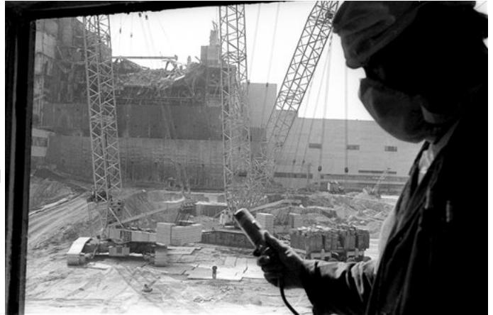
FILE In this 1986 photo, a Chernobyl nuclear power plant worker holding a dosimeter to measure radiation level is seen against the background of a sarcophagus under construction over the 4th destroyed reactor, Ukraine. On May 12, 1986, more than two weeks after the explosion, the leading Soviet daily newspaper Pravda published its first photograph from the site for the first time, shot three days earlier from a helicopter. The Chernobyl nuclear power plant explosion was only about 60 miles from photographer Efrem Lukatsky's home, but he didn't learn about it until the next morning from a neighbor. Only a few photographers were allowed to cover the destroyed reactor and desperate cleanup efforts, and all of them paid for it with their health. I went a few months later, and have returned dozens of times. (AP Photo/Volodymyr Repik)
